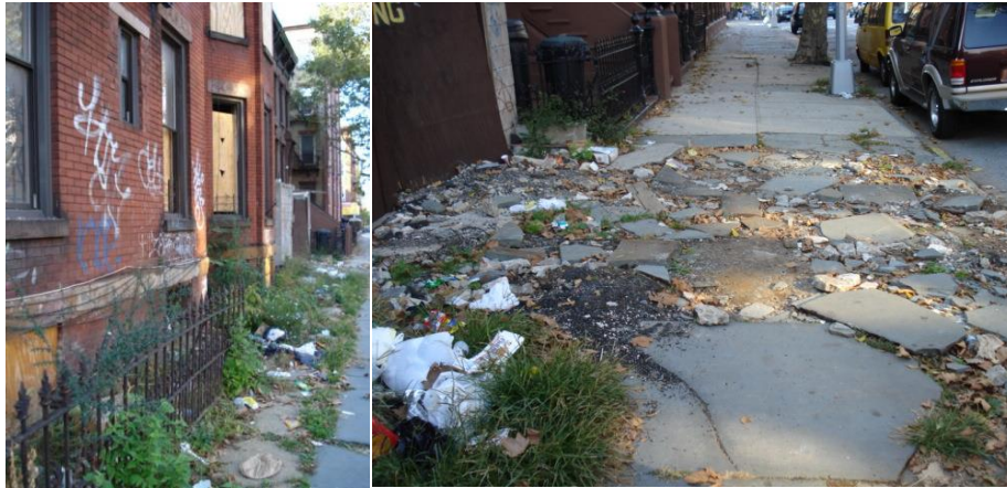
Abandoned building and severely cracked street in Bedford Stuyvesant, Brooklyn Images courtesy of bedstuyblog.com
