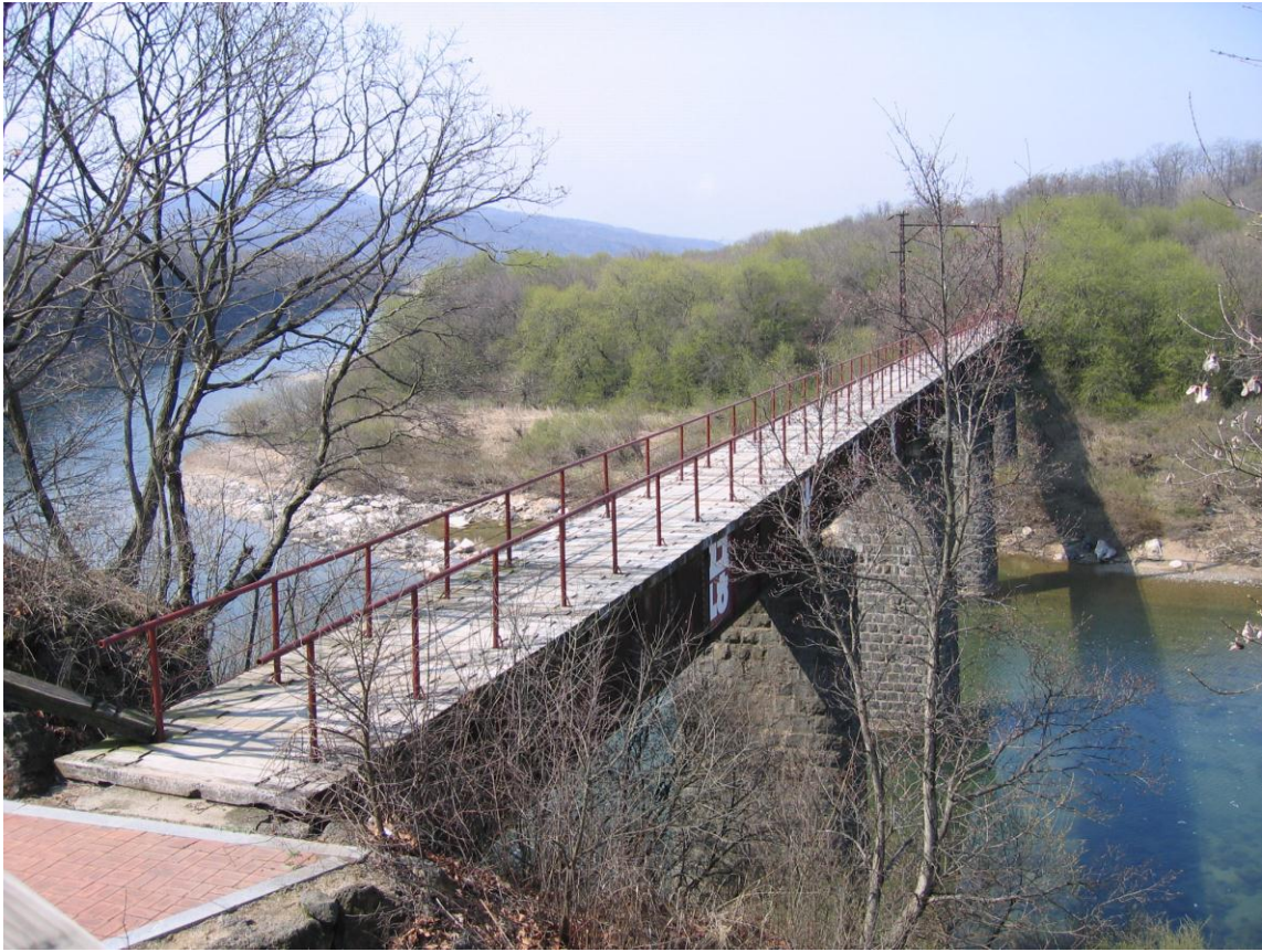
Mt. Keumgang Electrical Railway Bridge, Cheorwon, South Korea
